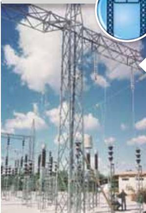
We manufacture a variety of outdoor electrical substation structures, including lattice, tubular and wide-flange steel support designs. Experience and knowledge regarding the use of these structures are essential as fabrication often utilizes complex welding processes. From in-service deflection limits to special grounding requirements, we also understand the needs of transmission line termination structures.
