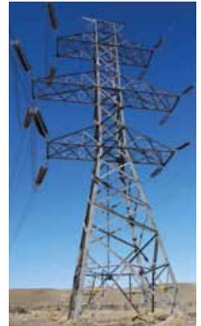
*Vertical dead end, 500/230 kV, double circuit*
