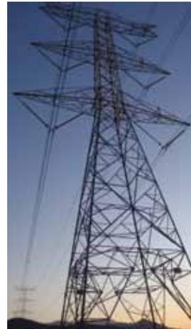
*Vertical, 400 kV, double circuit*
